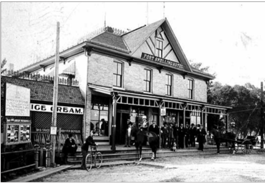
The Fort Snelling Hotel, West Seventh at Boulevard, was built by John Hammes from 1884 to 1886 at the end of the Fort Snelling bridge across from the Fort. It was successively owned by George T. Harris Saloon with its Ladies Waiting Room Restaurant (1887-1910); Nels Christ Johnson (1911-15); John P Kirk (1918); Einer M. Johnson (1919-20); Louise Sattler (1921-24). 1898 image MNHS
