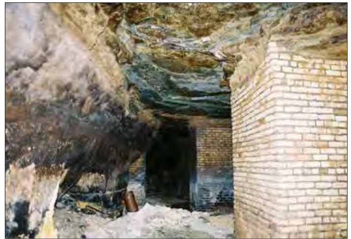
Stahlman’s cellerage. 2006 photo Andrew Hine
