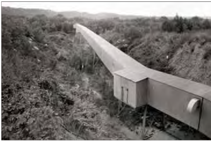
Archer Daniel grain conveyor from the terminal to the barges on the Mississippi River in its natural state before Shepard Road was built. 1958 photo RCHS.
