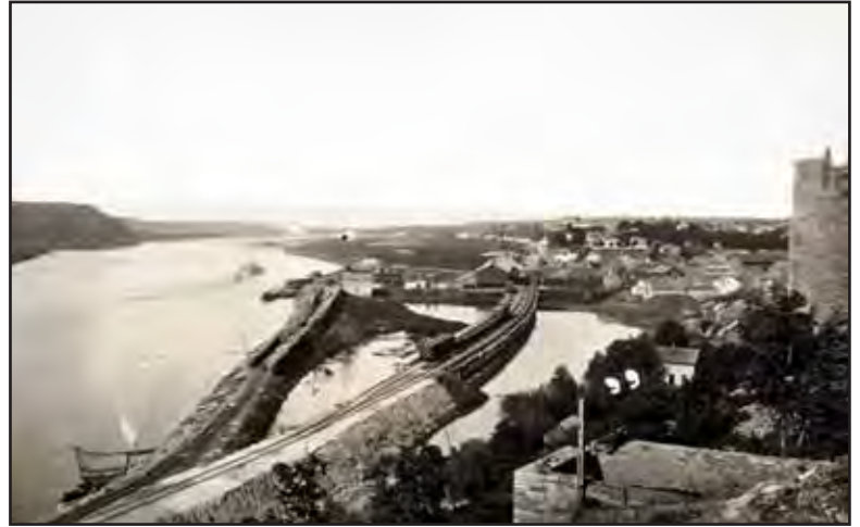
In 1873 the Upper Levee extended to Randolph and the river's flood plain had yet to be filled in, with railroad tracks built on trestles above. 1873 Bromley photo MNHS
