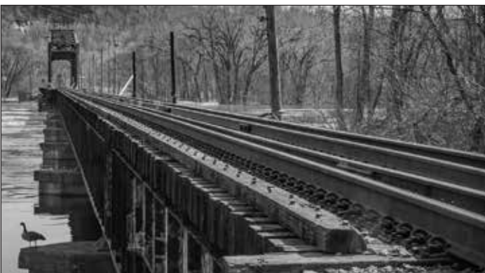
Omaha Swingspan Railroad Bridge. 2019 photo Craig Johnson
