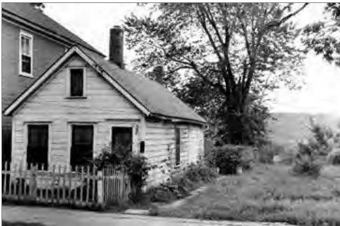
In the 1895 census, Connie Aubert lived alone at 764 Butternut. It was built about 1884. When wrecked, it was heated by an oil stove and had a “water closet” and sink. Photo compliments RCHS.
