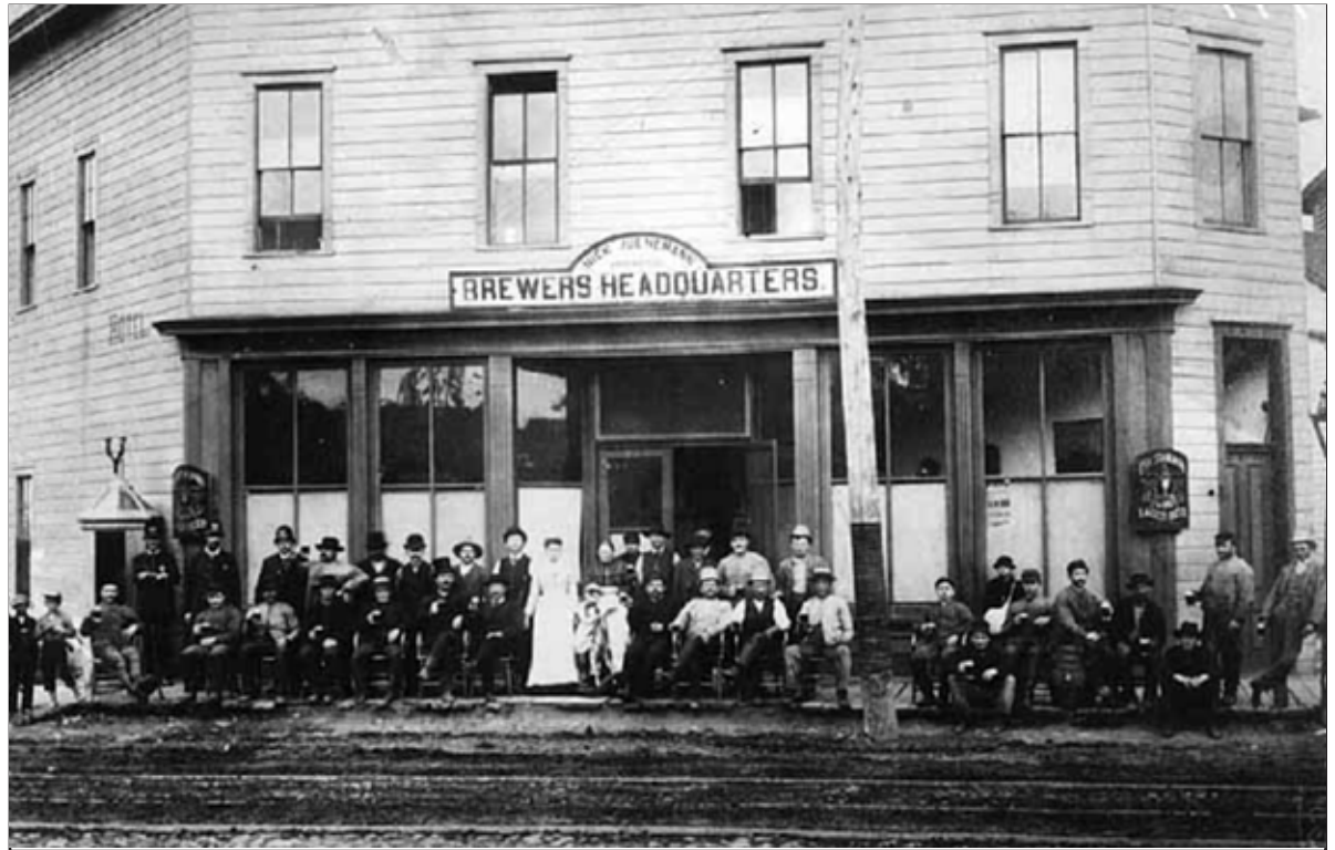
904 West 7th Street: Nicholas Juenemann's Hotel and Saloon: Brewers Headquarters. As related by Harry Hoenck in the St. Paul Pioneer Press March 3, 1963: Christopher Stahlman's Cave Brewery (predecessor of Schmidt Brewery) was behind the hotel; he is leaning against the lamppost at right. The lamppost was wrapped in wire to discourage horses tied to it, as horses loved to gnaw the wood. Unpaved Seventh Street had a horse-car line at the time. Hoenck's father, William Hoenck (1853-1919), a Prussian immigrant, is the third policeman in the back-left row. 1889 image: MNHS.
