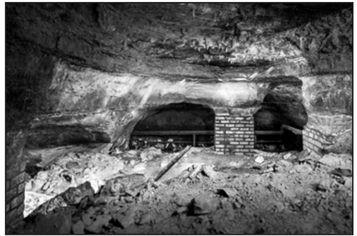
Between the ice chute and the back of the north section of the cellars, a little pillar shows where a room used to be. The space seems to be the last point of expansion in Schmidt’s cave cellerage—last carved in the mid-1800s. Image Dan Turner, Substreet.org
